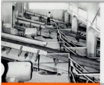
Above: Three conveyors feed ore into the standard cone-crushers.
