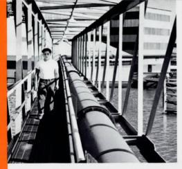
A Kennecott workman walks over bridge-like structure alongside big pipe through which tailings flow to center of the 325-footdiameter Tailings Thickener at Hayden.
