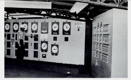
The control center for the Moly Plant is the heart of the operation. Direct reading meters allow the operator to constantly check and adjust the flow of material from one phase to another.
