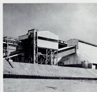
The smaller of the two buildings above is the "Transfer House" that receives up to 1800 tons of ore each hour from Crusher, and deposits it in the larger building which is Fine Ore Storage Bin. This tent-like steel and concrete building is longer than a football field and has ore storage capacity of 28,000 tons.
