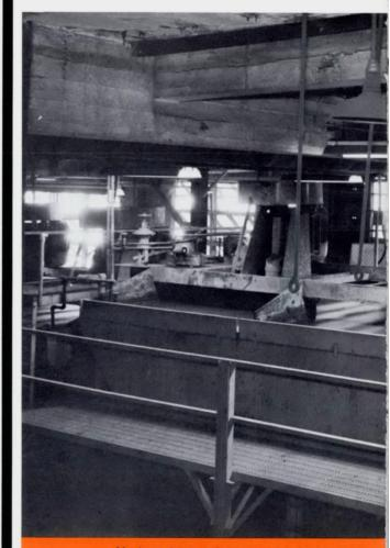
Modern, high-volume mechanical flotation cells have recently been installed in the Hayden Concentrator replacing older, smaller air flotation cells. Five, 15-cell rows of these
