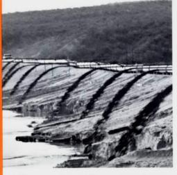
Tailings pour into a 900-acre disposal area. A crew of 13 men, two drag lines, three dozers and two scrapers are required to build dikes, maintain and patrol them around the clock. Water in the pond is siphoned off and sent back to the mill for re-use. Photo at right: night dike-walker.
