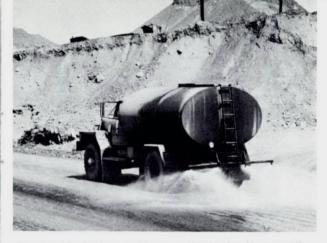
To provide better working conditions for Kennecott's workmen — and to minimize abrasive wear on equipment — dust is controlled by frequently sprinkling the truck haulage roads with water.
