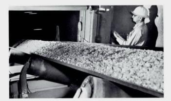
"Weighing a mountain in motion." As it leaves the Crusher Building on conveyor belt a "weightometer" keeps a record of the ore tonnage produced by each eight-hour shift.
