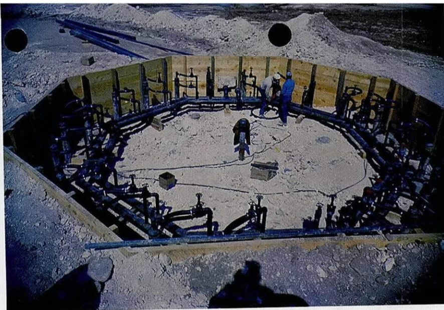
Nash Draw ore hoisting shaft location showing refrigerant manifolds and freeze well locations prior to commencement of sinking operations.
