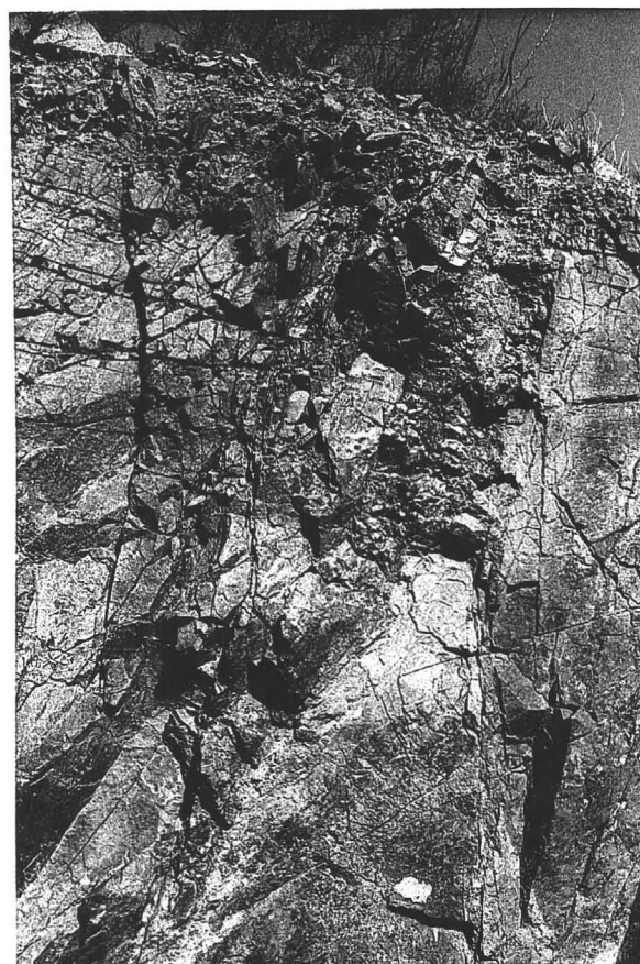
(16) (Neg.#19) East Wall of Caved Main Adit Portal.
