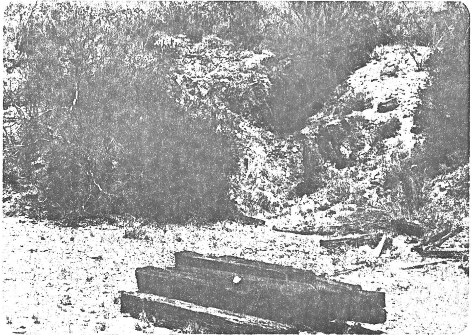
Entrance to principal shaft that descended some 400 feet.
