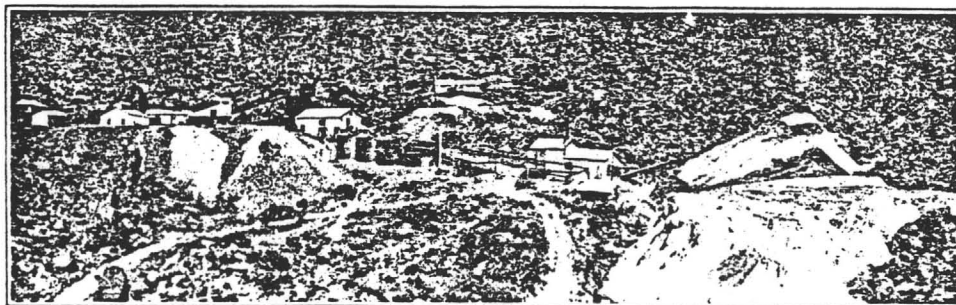
A general view of the Liberty Hills Gold Mines, Ltd. From left to right are shown the office, headframe and hoist house, crushing and conveying equipment, cyanide plant, precipitation plant, and tailings.
