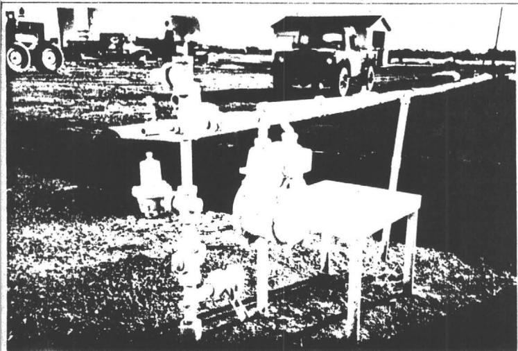
HIGH PRESSURE GAS REGULATOR
