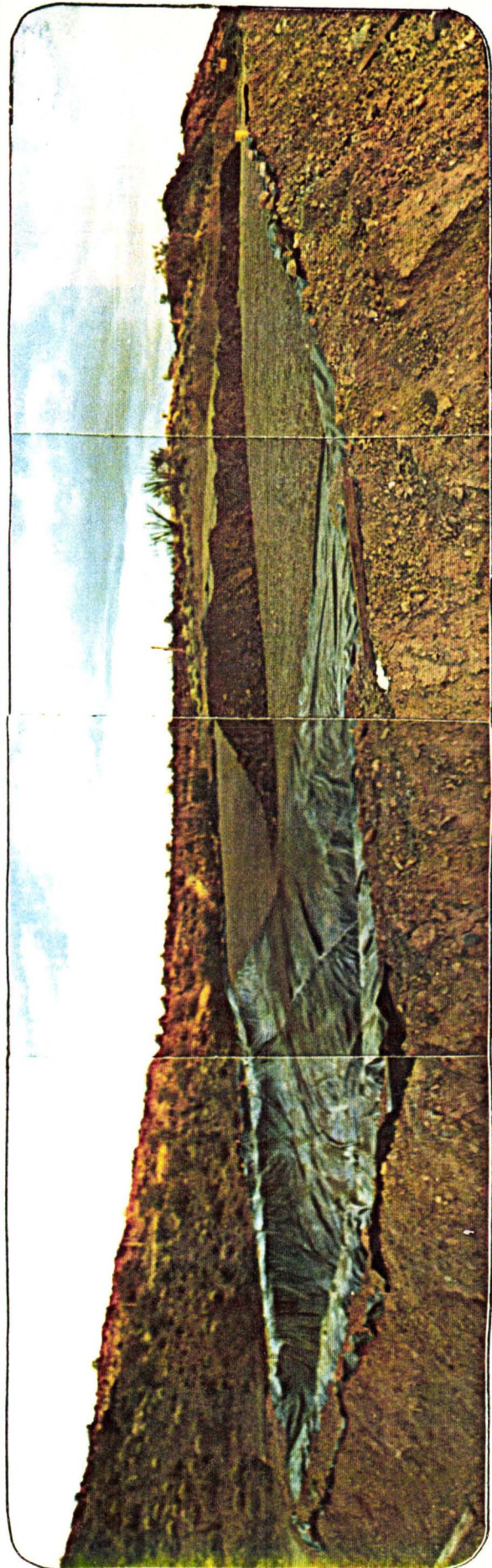
Loading the pad with ore
