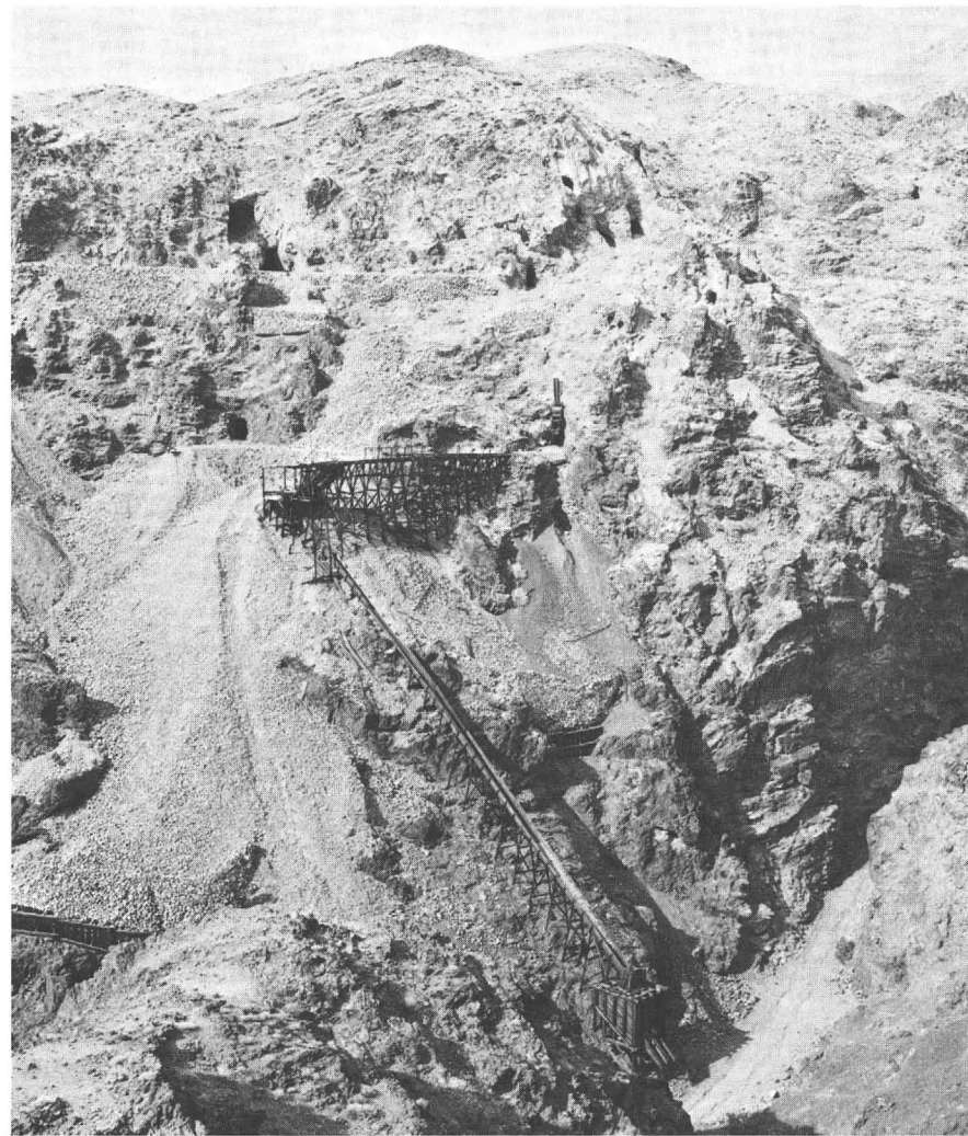
View west-northwest in 1951 shows old workings of Odessa silver mine, on west side of Odessa Canyon, East Calico, mined principally from 1882 to 1896. Rugged topography is cut in andesite. Ubiquitous, gopher-like workings resulted from expedient mining of near-surface, "bonanza" deposits. Photo by O. A. Russell, Yermo.
