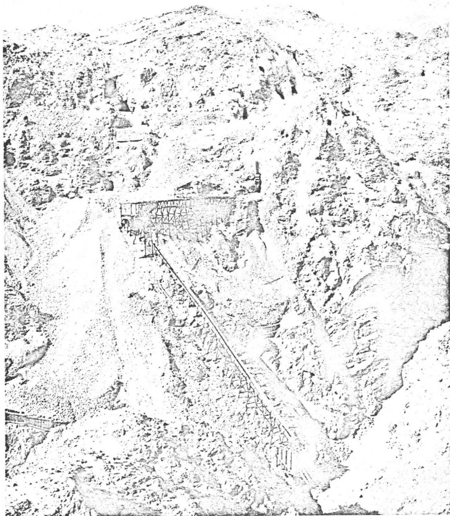
View west-northwest in 1951 shows old workings of Odessa silver mine, on west side of Odessa Canyon, East Calico, mined principally from 1882 to 1896. Rugged topography is cut in andesite. Ubiquitous, gopher-like workings resulted from expedient mining of near-surface, "bonanza" deposits. Photo by O. A. Russell, Yermo.
