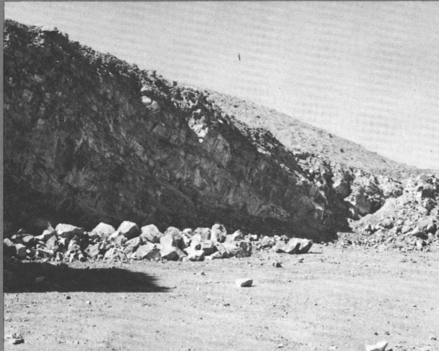
Photo 14 (top). West face of Quarry 12 of Southwestern Portland Cement Company, showing gently dipping, platy character of the limestone of map unit VIIA. Quarry 12 was one of the principal sources of limestone for the Victorville plant from 1938 to about 1951. Photo, March 1960.
