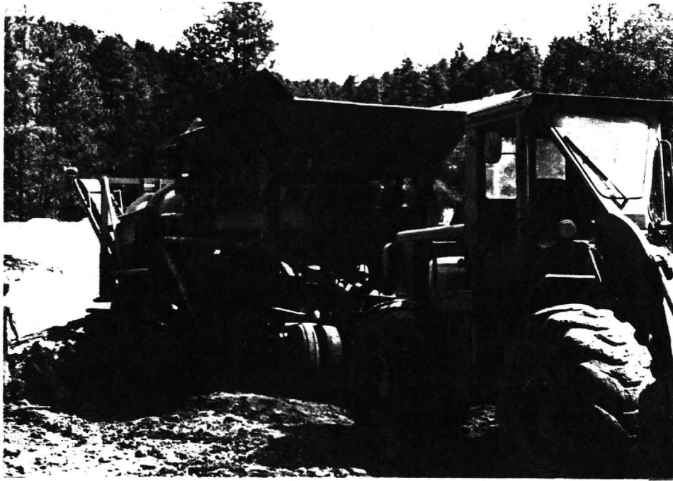
MOVING THE TROMMEL & GRIZZLY INTO POSITION
