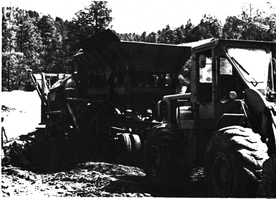
MOVING THE TROMMEL & GRIZZLY INTO POSITION
