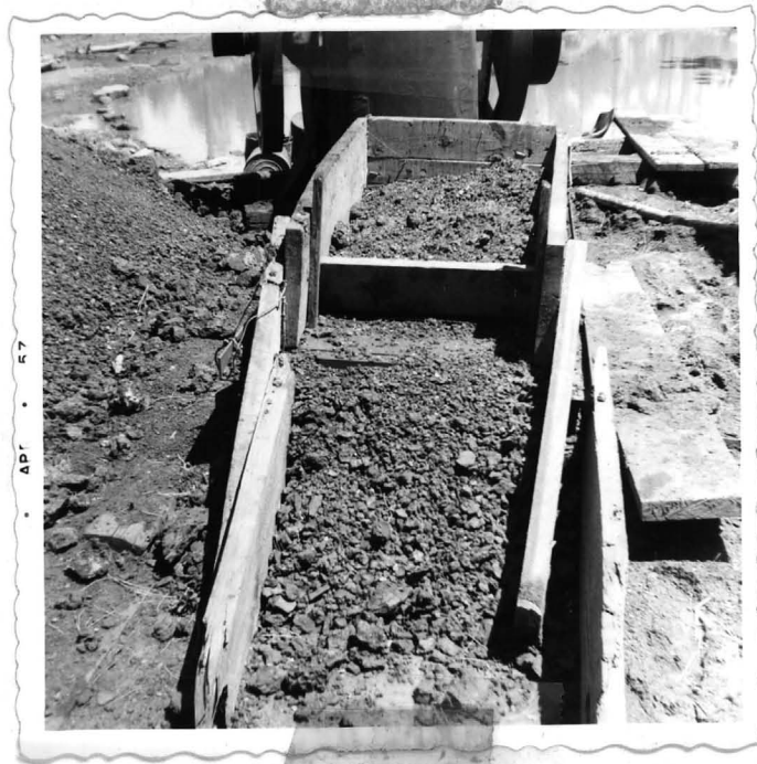
Photo 5-Shows front end of stationary \frac{1}{4} " screen and box. Owner hose-washes material at left in screen box, leaving coarse product in front end.
