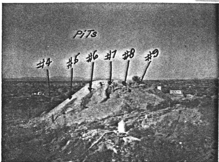
March 11, 1981 - SE side of Conical Dump Showing Backhoe Pits 5, 6, 7, 8 & 9. 12:00 Noon.
