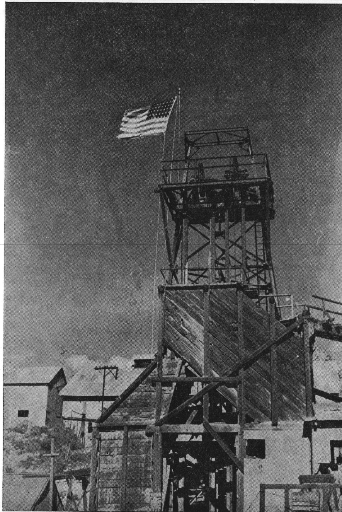
Steel Headframe and Ore Bins at Collar of 1400 foot vertical shaft at Tennessee Mine.
