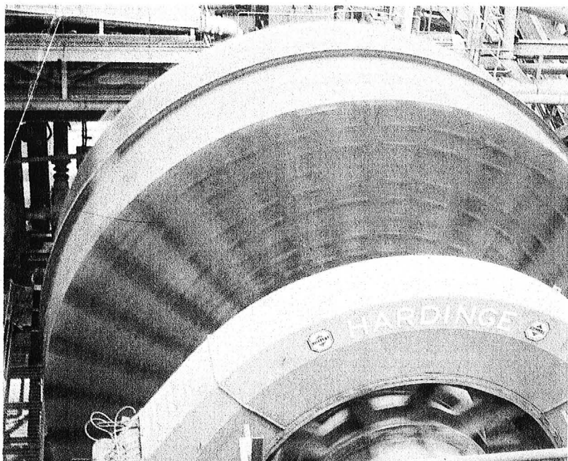
(2) Hardinge 32' x 12' Autogenous Mills, Twin 3400 H.P. Motor, 4160 volt
