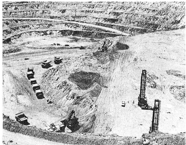
Many operations underway simultaneously in the pit. At right, a survey crew is dwarfed by two rigs drilling blast holes. In the background, left of center, another crew loads explosives and in the foreground, an electric shovel takes three or four bites to load a 100-ton dump truck with ore.
