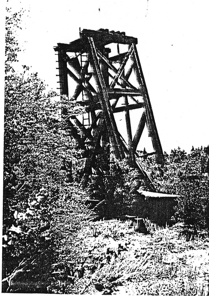
Figures 5 and 6: Tiger Mine headframe and ore bin/mill foundation. Note granitic country rock.
