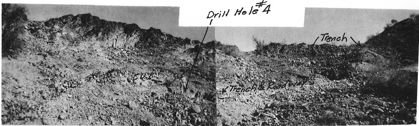
This shows trenching and cut work as well as road recently graded on westerly side of Outcrop Hill. Figure in picture shows location of Drill Hole 4. See assay logs of drill holes and accompanying map.
