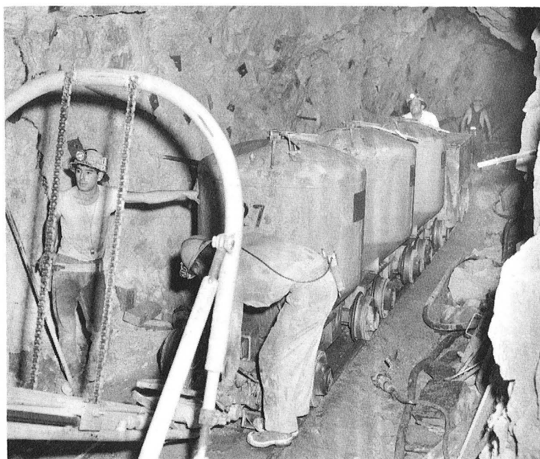
FIGURE 41. - Coupling Placer Pots to Slickline.
