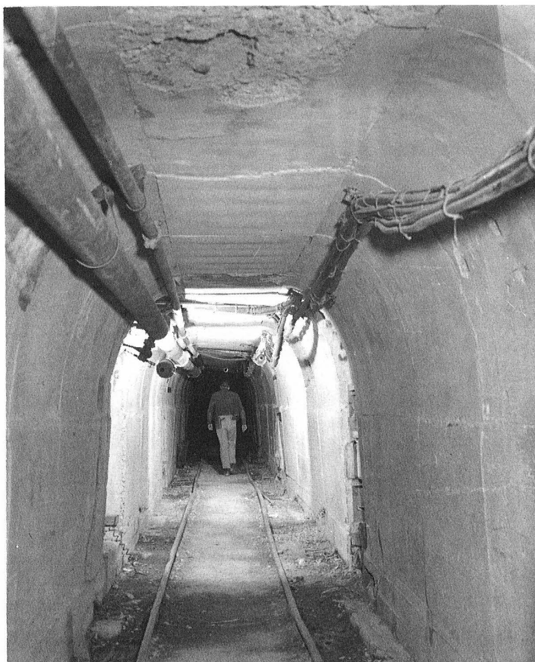
FIGURE 38. - Concrete-Lined Panel-Fringe Drift.
