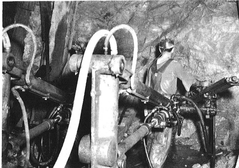
FIGURE 17. - Two-Machine Jumbo at Face of Drift.
