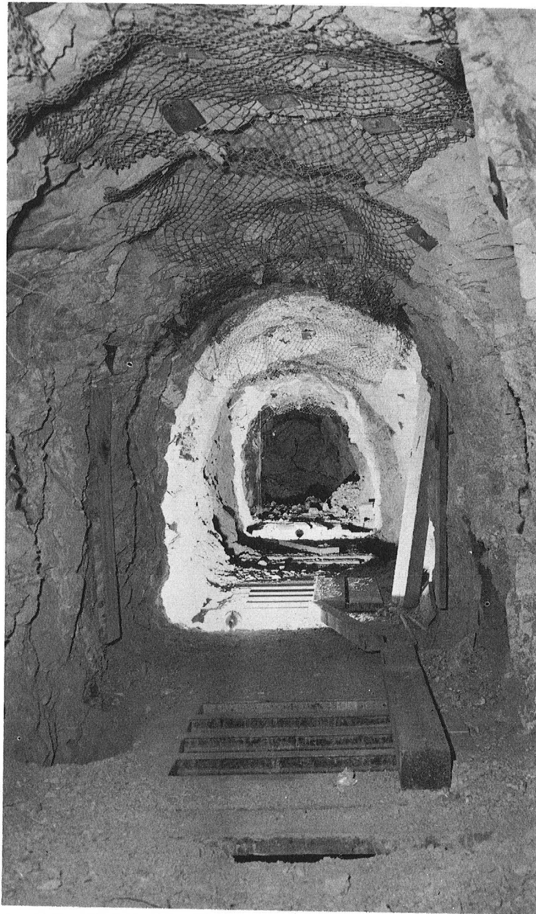
FIGURE 27. - Grizzly Drift Prior to Concreting.
