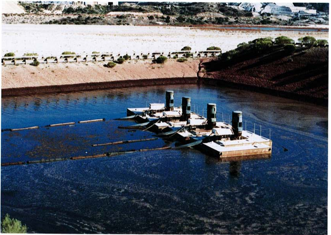
Copper bearing solution from the heap is collected in pregnant leach solution ponds.
