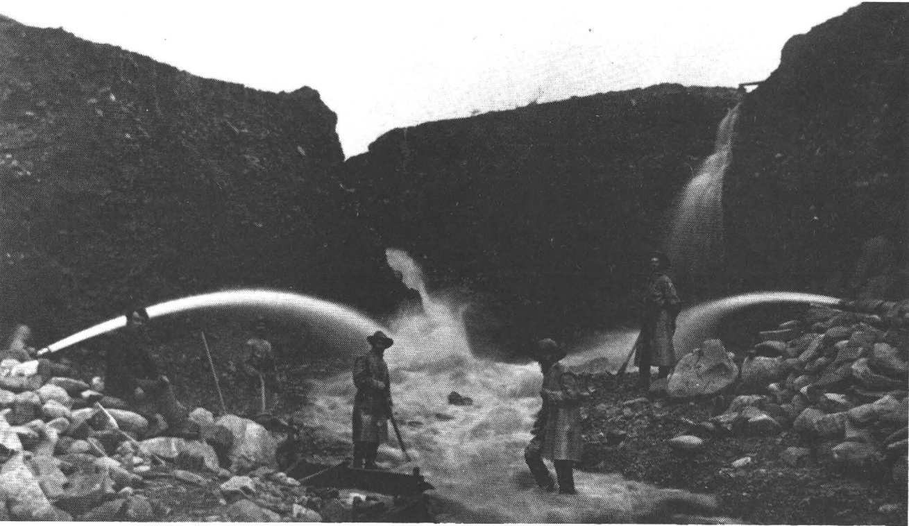
Figure 5. Hydraulic placer operation on Lynx Creek, circa 1890. Photo courtesy of Sharlot Hall Museum.
