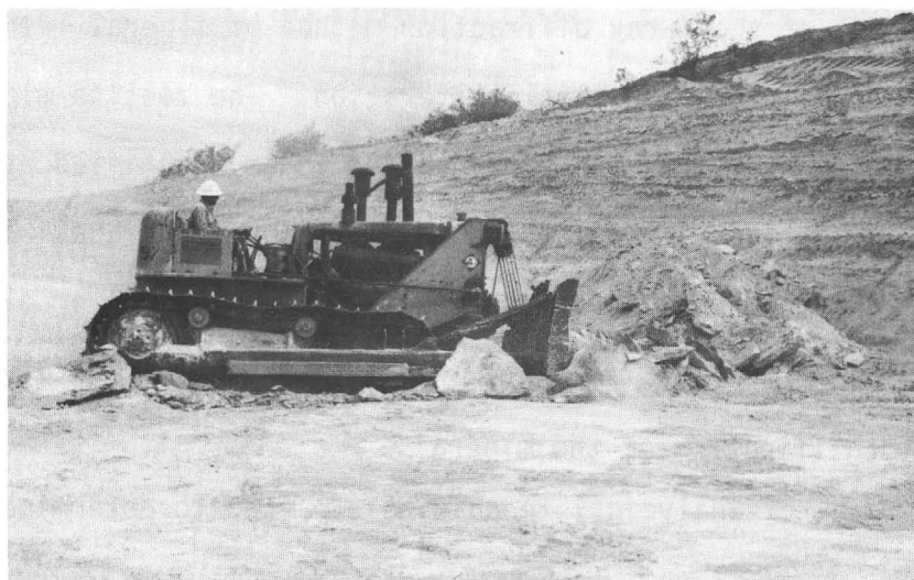
EZ 185 - Cleaning Sandstone Overlying the Chabazite Bed
