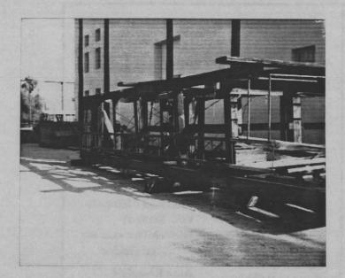
One of the last surviving wooden headframes, built in 1917, lies waiting for assemble after being transported from Phelps Dodge's Boras mine in Bisbee.
