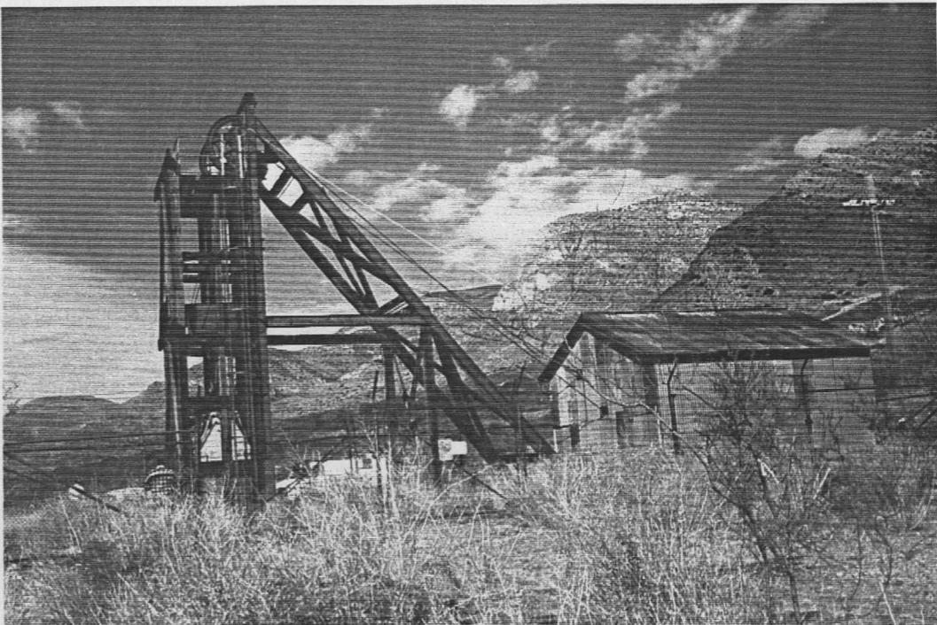
The Boras headframe, a gift from the Phelps Dodge Corporation, will be dismantled to allow shipment from Bisbee to Phoenix. APS is generously providing transportation to the museum. It will be reerected west of the Museum along with the hoist and hoist house. The cages, turn sheets, and the controls will also be salvaged and moved to the museum.
