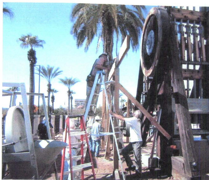
Volunteers start construction of the operator and feeding chute platform for the stamp mill in front of the Museum.
