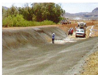
Stabilization wall construction in lower 3-4 channel.
