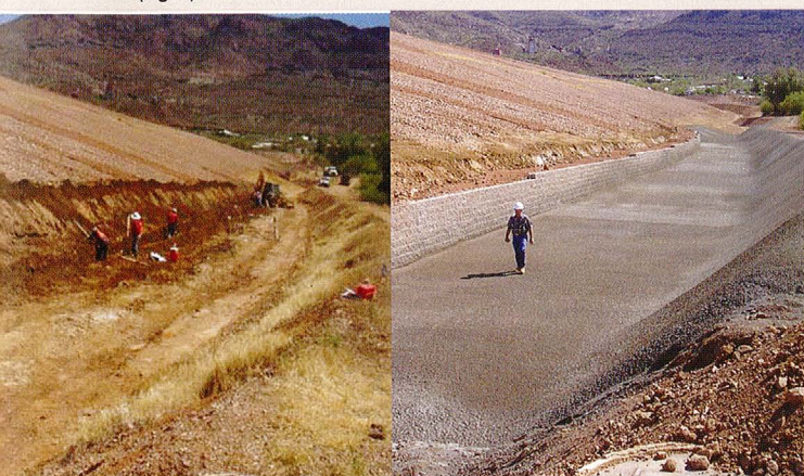
(left) Before: Pre-construction view. (right) After: Stabilization wall construction in lower 3-4 channel.
