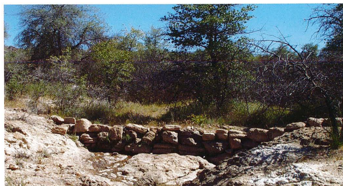
Example of a dry-laid masonry "check dam" with three courses of stone
