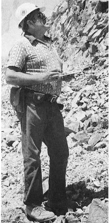
"Mapping a bench" is a routine, but important task of the Geology Department. Here, Neil A. Gambell, division geologist, with clipboard in hand and the tools of his profession attached to his belt, walks along a deserted bench in the silicate area making notes, collecting samples and leaving spray-paint numbers on the rock faces to guide the department survey crew when they return to the scene to do the final mapping.
