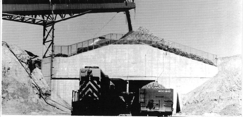
The "ore drag" starts at the loading tunnels under the open air stockpile at the primary crusher in the Mines Plant. Half of the 55-to 60-car train has been loaded from the tunnel on the right and on the left the RMD locomotive is slowly pulling the second half of the train through the loading tunnel. When all cars are loaded, the train will start its journey to Ray Junction.
