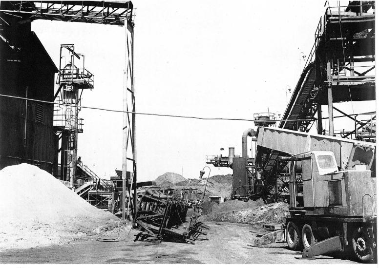
This is a dramatic example of work done by Smelter Maintenance during the vacation shutdown. An important conveyor had to be reconstructed and here's the job at its mid-point. That missing section of the high conveyor, seen on the ground, was later used to fill the gap and connect the two areas.
