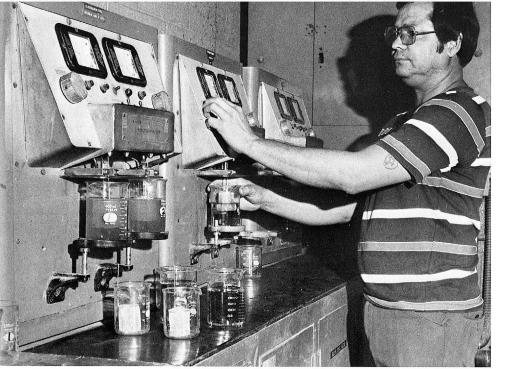
These Electro-Analyzers in the Mines Plant Quality Control Laboratory are probably the hardest working pieces of equipment at that location. Quality Control Technician Jesus G. Olmos, Jr. is shown running an assay to determine the purity of copper precipitate being shipped to the Nevada Mines Division.
