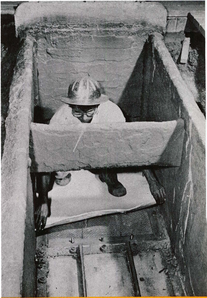
This Kennecott workman in the L-P-F Building at Hayden is installing a new canvas "matt" in the bottom of one of a battery of trough-like Flotation Cells. The air is pumped through strong metal screen beneath canvas.
