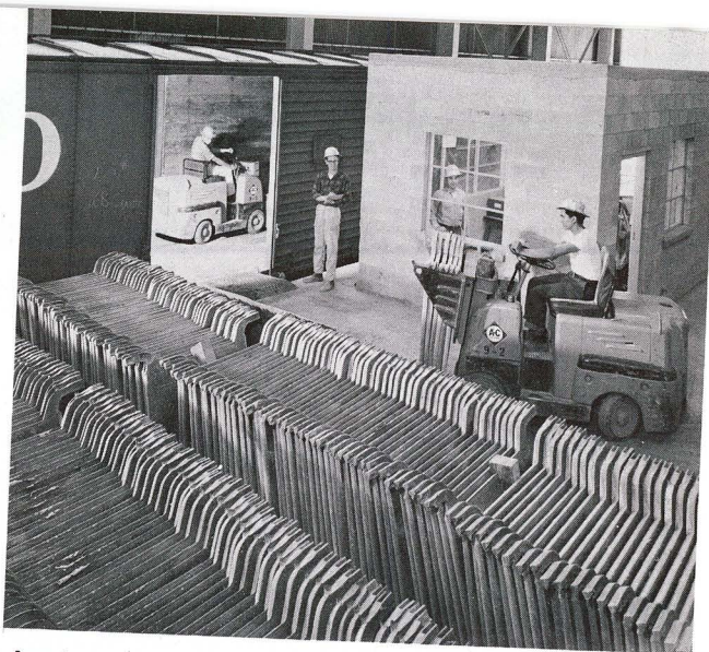
Anodes, after being approved by Quality Control, are picked up, several at a time, by fork-lift trucks and loaded in box-cars for shipment to Kennecott Refining Corporation in Anne Arundel County, Maryland, for electrolytic refining.
