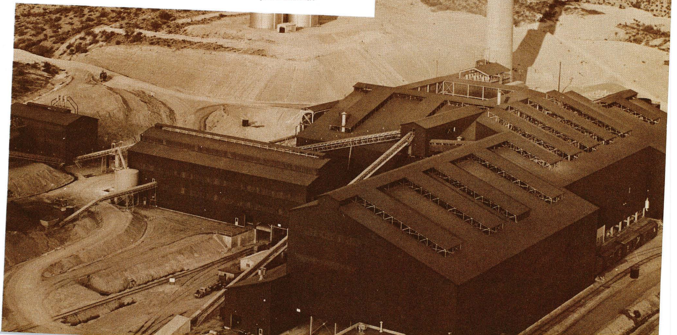
Aerial photo shows Smelter Building and supporting facilities of Kennecott Copper Corporation's Ray Mines Division in Hayden, Arizona. For each 700-pound anode produced here, 90,000 pounds of copper ore must be processed.
