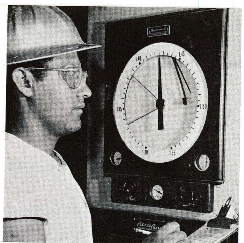
This dial records the amount of "tailings" handled by Water Reclamation Pond, and other information about system's operation. Saving: 4½-million gallons per day.
