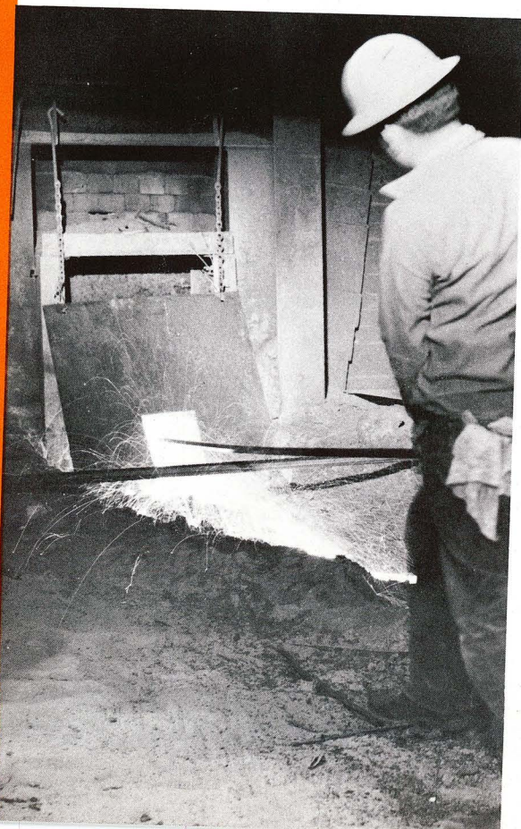
Right: 20 tons of matte copper is moved into the converter aisle by the workman pictured, who is operating the control of the matte car. The ladle will be lifted from the car and taken to one of the three huge converter furnaces.
