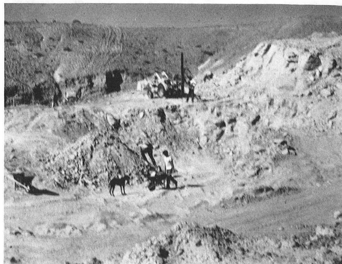
Mining at the Charlie Huskon No. 3 open pit in the Cameron area, April 1966. Uranium here is in sands and shales of the Triassic-age Chinle Formation. Petrified wood in the sediments is especially uranium rich. Photo by W. Chenoweth, Dept. of Energy.
