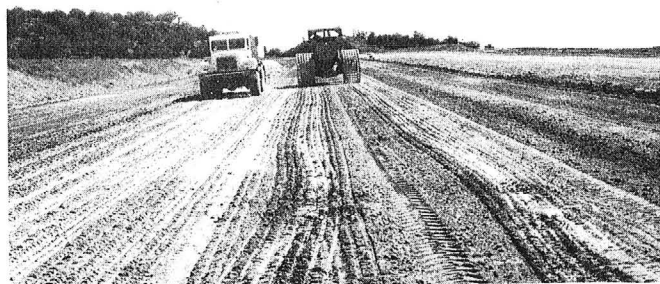
The hydrated lime road was smoothed with grader and compacted with Grid roller.
