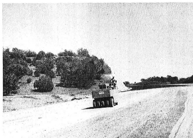
Rubber tire roller did the final compaction.
