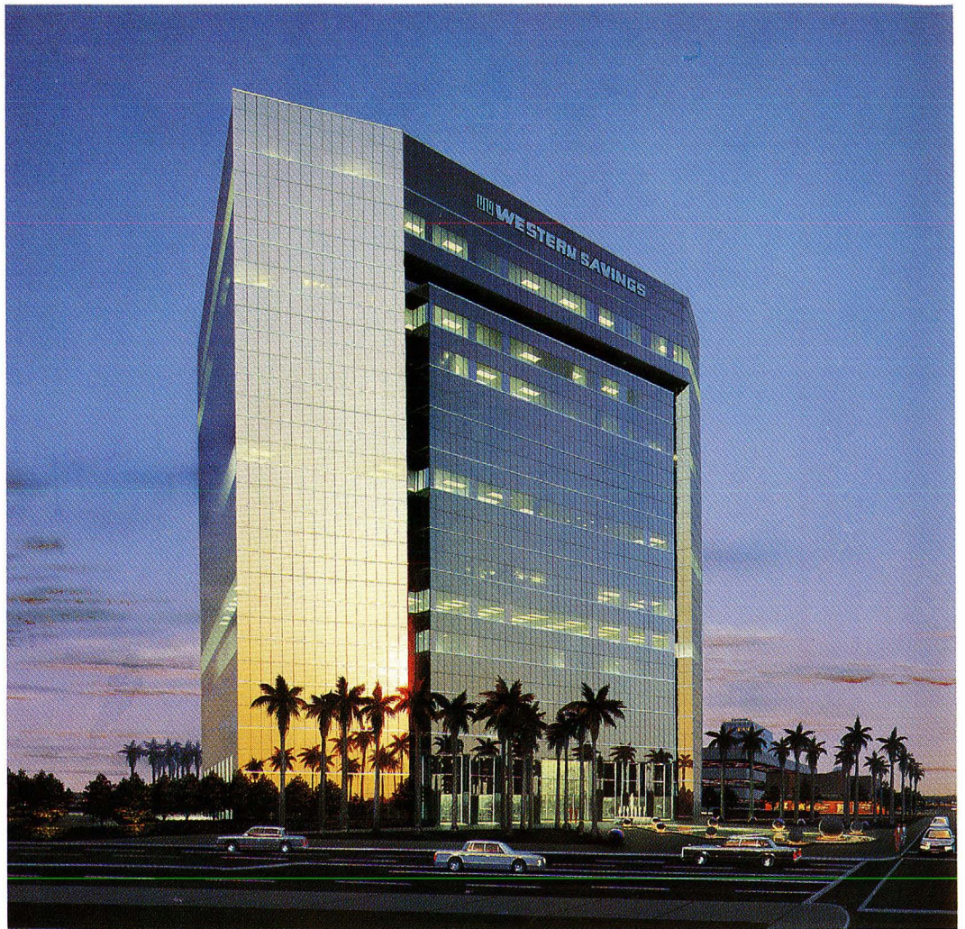
Western Savings Financial Plaza, developed by the Wolfswinkle Group, Sundt Corp., General Contractor
