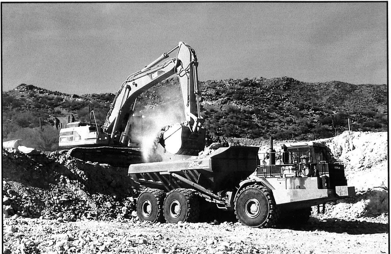
Mining Central Pit
