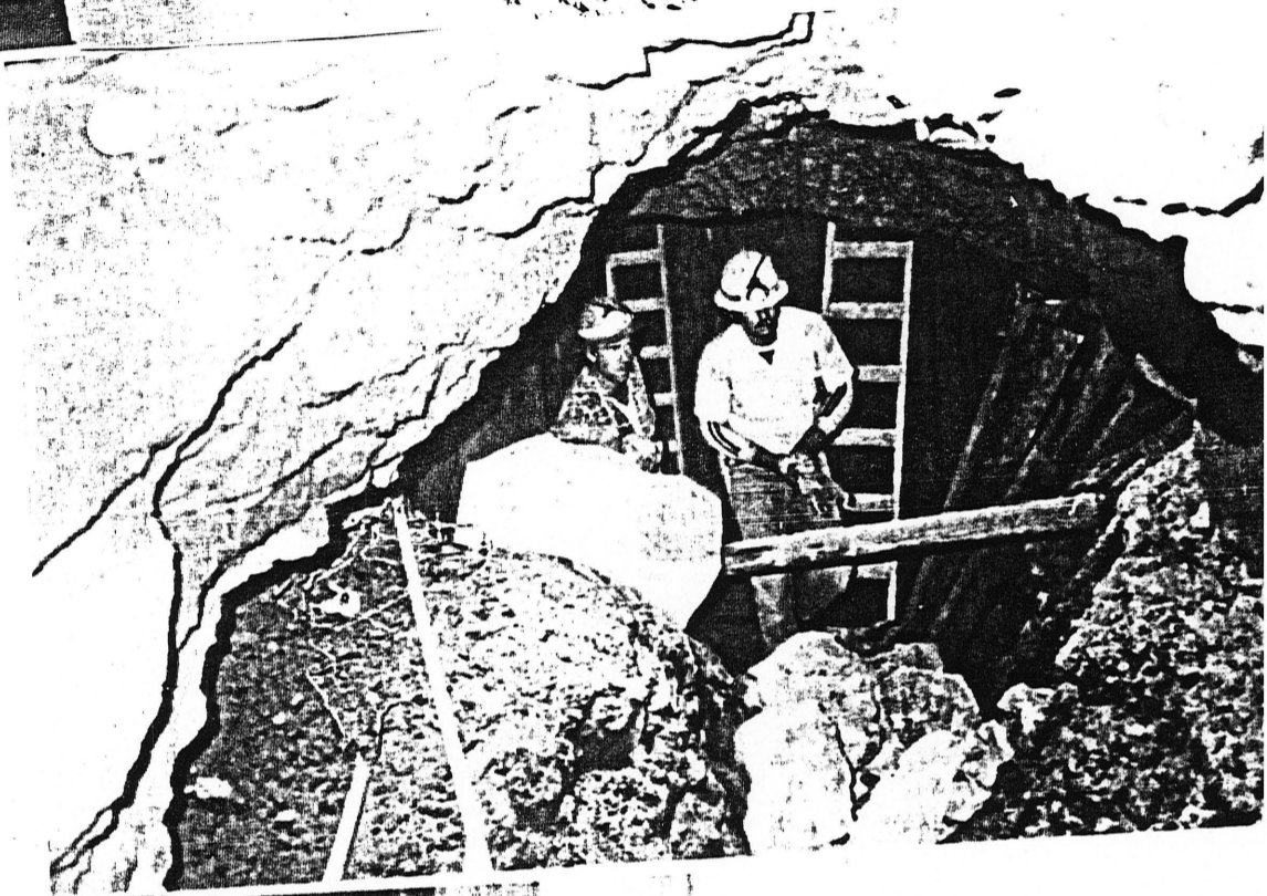
OVER 3000 TONS OF MUCK HAD TO BE CLEARED.
