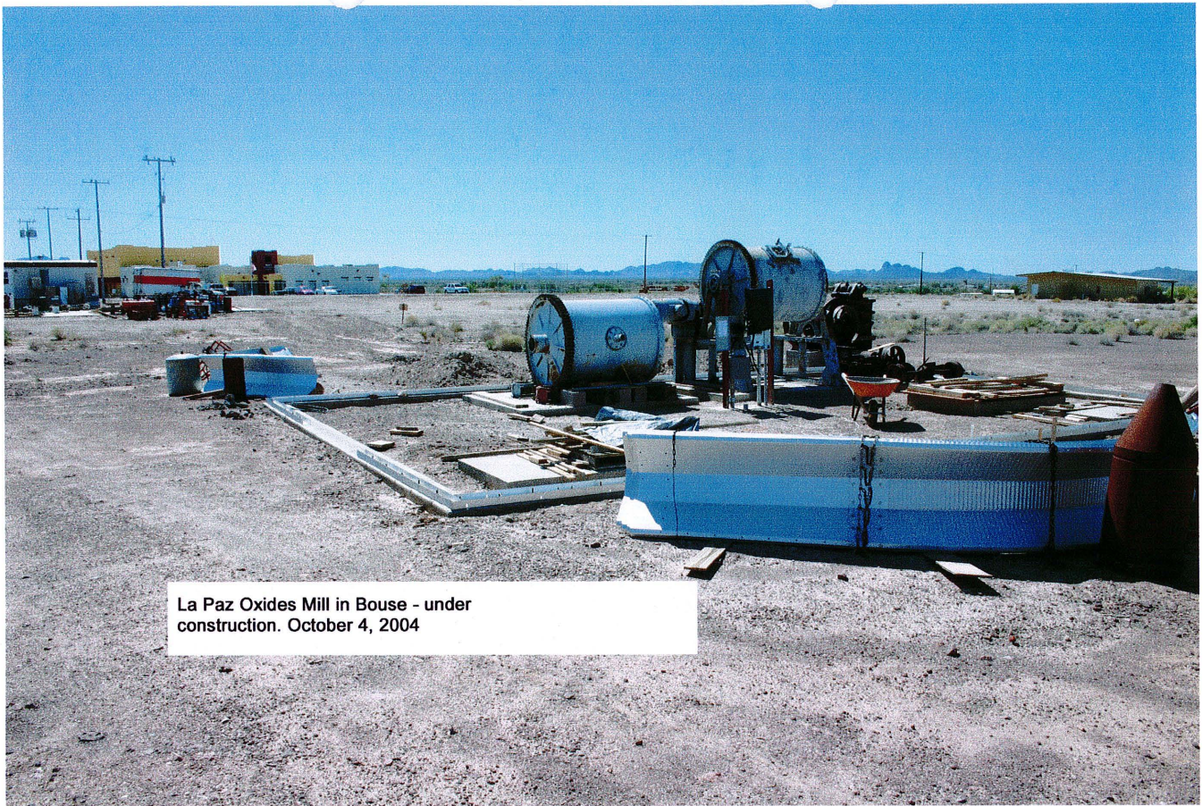
Patterson ball mill (on stand) and Burrstone mill (both are 4' Dia. X 5') for La Paz Oxides mill. Footings and mill foundations are complete. October 4, 2004.
