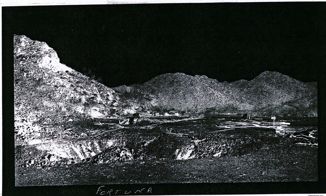
CAVED-IN DUMP IN FOREGROUND. DEEP SHAFT COLLAR UNDER TIMBERS AT MIDDLE RIGHT.
