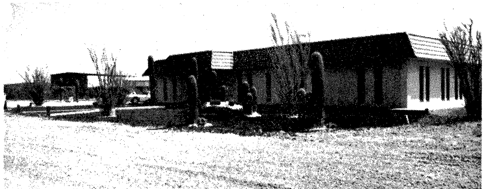
Office facilities are located on-site near the main plant building.
