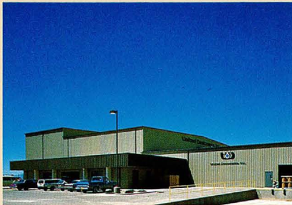
The modern plant in Belen, NM was built in 1983.
