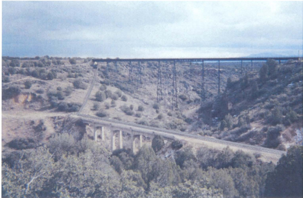
Figure 2-5. Approximate proposed conveyor alignment (shown in gray) across Hell Canyon Bridge, up the hillside and under the railroad trestle. View to the southeast.
