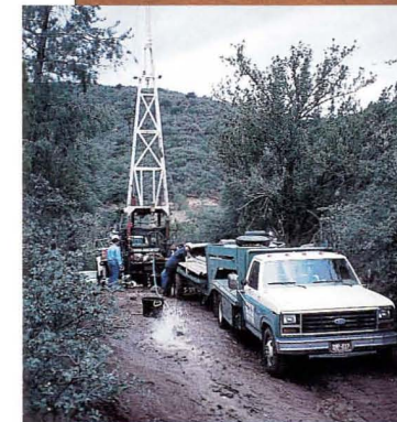
Pump test drilling.
