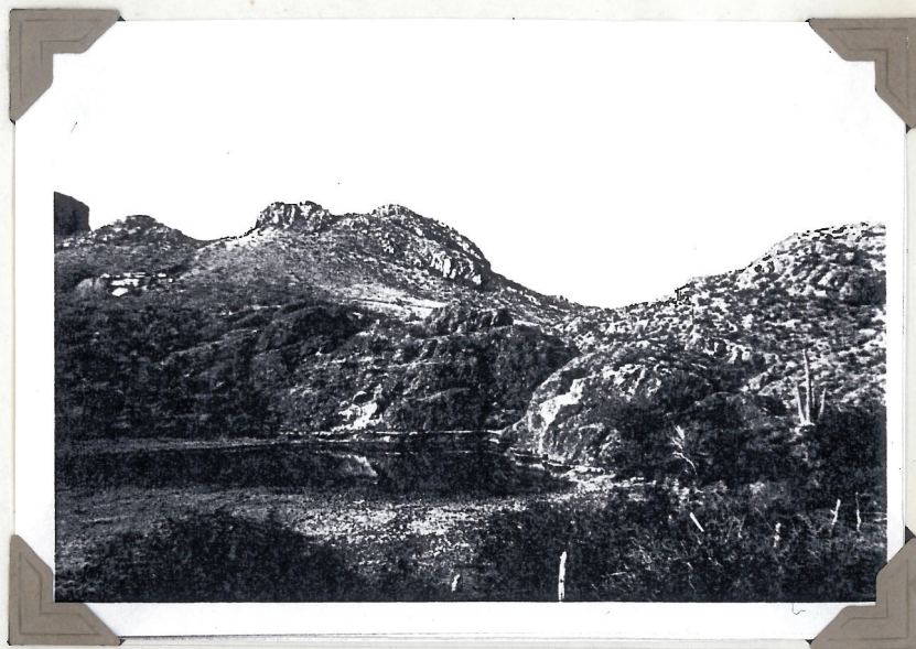
(b) 2. Allison Dam and Reservoir, looking northwesterly.
