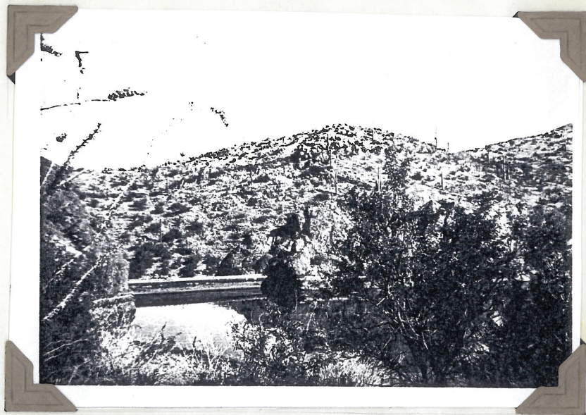
(b) 1. Allison Dam and Reservoir, looking southwesterly.
