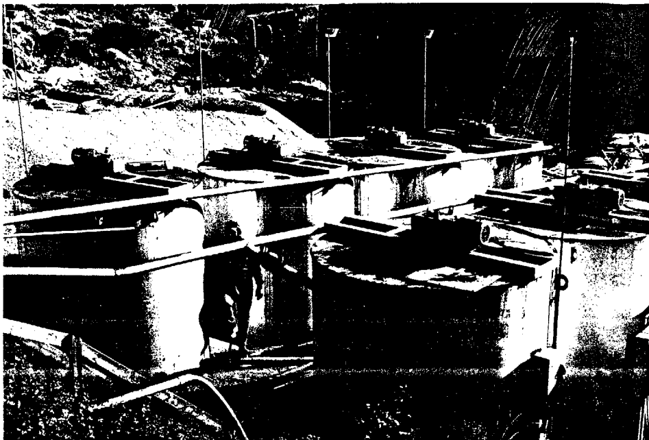
AQUISITION MILL SITE SLURRY AGITATION TANKS
