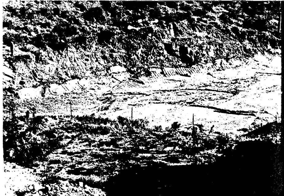
SITE OF LEACH PAD 26,000 TONS CAPACITY WHEN COMPLETED
